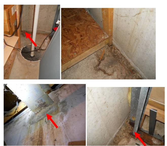
• The floor near the water softener in the basement is wet. This maybe from condensation.
