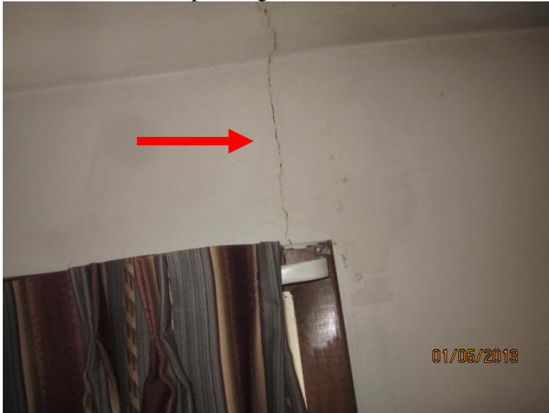
Bedroom cracks and patching
