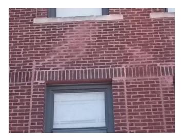
• The top of the building on the west side has been parged with mortar. This type of repair tends to crack off in time. So far, the work is in satisfactory condition. There may have been a small roof or façade here at one time.
