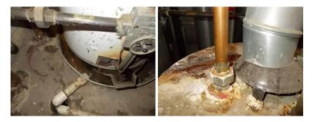
• There are moisture stains at the furnace vent at 5221, unit 2B which means it is not drafting properly. This can be a dangerous carbon monoxide hazard. The room for this furnace and water heater does not have adequate air for combustion of the gas appliances so this may be part of the problem. Have a licensed HVAC professional check this out.
