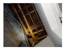
• The PVC furnace vent should have a continuous upward pitch otherwise it might have drafting and condensing problems.
