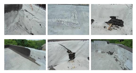
• The roof membrane is not firmly attached to the parapet walls because the parapet masonry is likely failing behind it. The parapet wall will likely need to be repaired and rebuilt around most of the perimeter of the building. This should be done in conjunction with the new roof installation. Consult a qualified mason.
