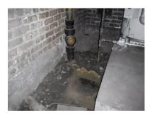
• The east basement shows signs of past flooding. There was a note on the wall concerning sewer backup. It is not uncommon for older to have hidden sewer problems. Drain pipes under the ground can leak attracting tree roots and other blockage problems. These types of problems can be latent so I recommend a TV scope of the underground drain/sewer by a licensed plumber to see if there are any issues.
